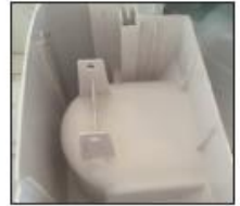
You can now access inside of water tank
